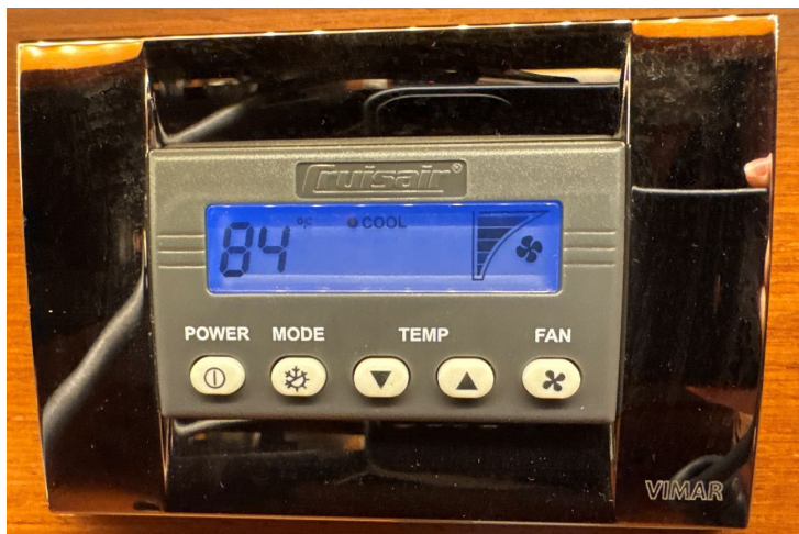
Cruisair A/C control panel — POWER, MODE (cool/heat), TEMP up/down, FAN speed
